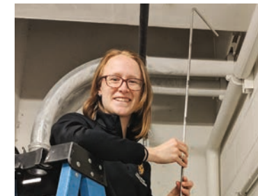
IES Senior Ansley Ostiguy (BA '19) uses a pitot tube to measure the air flow through the vent in Cuneo Hall.
